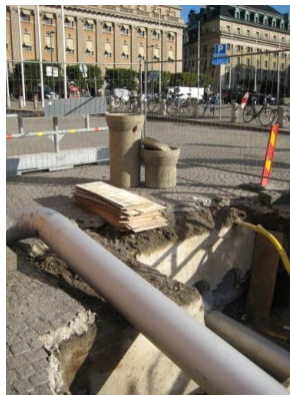
Unprotected type 304L drinking water pipe in the city centre of the Swedish capital Stockholm. Source: Euro Inox, Brussels (Belgium), www.euro-inox.org
