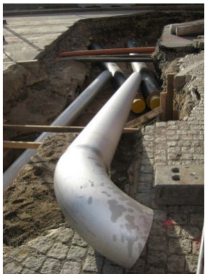
Unprotected type 304L drinking water pipe in the city centre of the Swedish capital Stockholm. Source: Euro Inox, Brussels (Belgium), www.euro-inox.org
